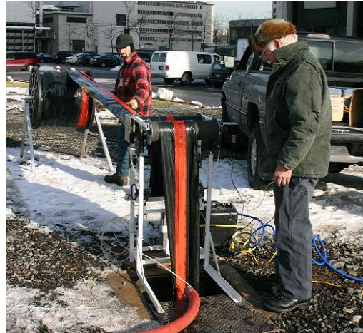
Fig. 7. The liner Profiling machine
