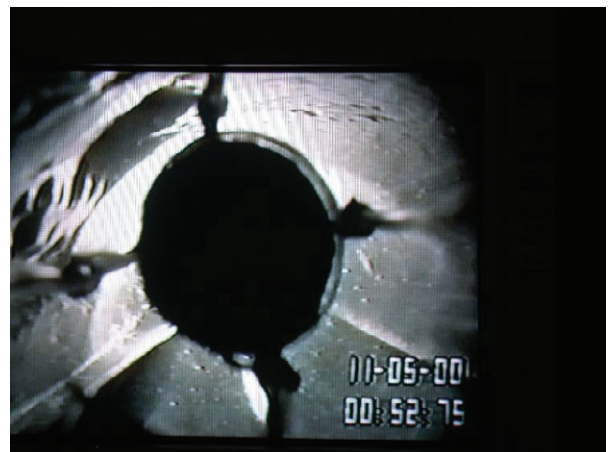
Figure 11. A borehole video snapshot of the interior of a 150 mm blank liner. The liner melds very well with the dolomite borehole wall, even over a ledge in the upper left corner of the photo. Individual vugs are visible behind the liner (top of photo). Packers cannot conform so easily to the borehole wall.
